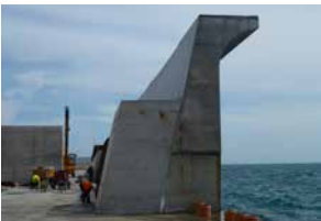
AUSTRALIA | Measurement of hydrodynamic forces on a loading platform
